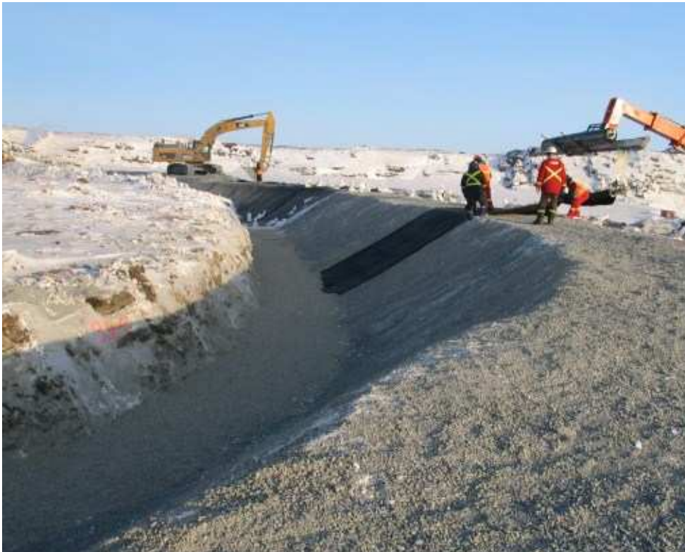
Photo 8: Layfield placing underliner from Sta 3+30 to Sta 3+80
