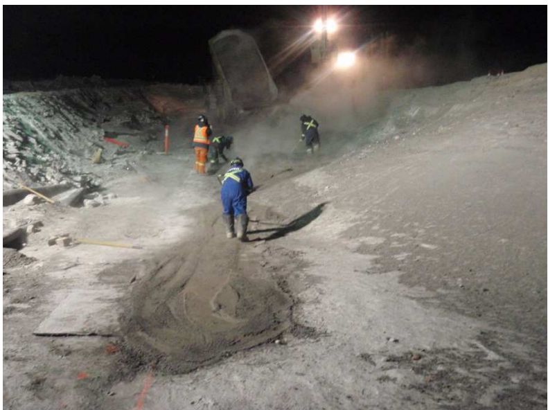
Photo 10: Labourers smoothing FCM in SE core area after packing with hand tamper
