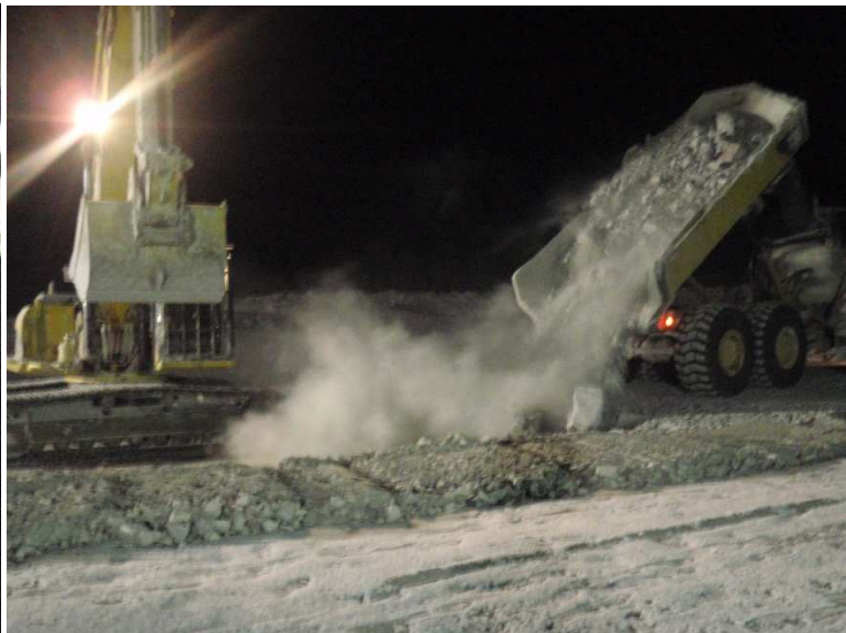
Photo 11: Excavator placing ROQ on downstream slope
