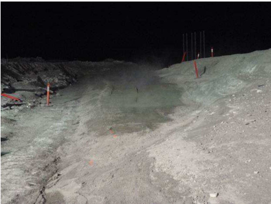
Photo 10 (with Acad Screenshot): ~ SW view of the area where placement along the SSE dam slope was completed on night shift. For reference a screenshot showing the as-built breaklines (as of March 10 th ) is provided. Note the indented almost 'U' shape underbuilt area of the SSE slope. This was the area of focus on tonight's nightshift.
