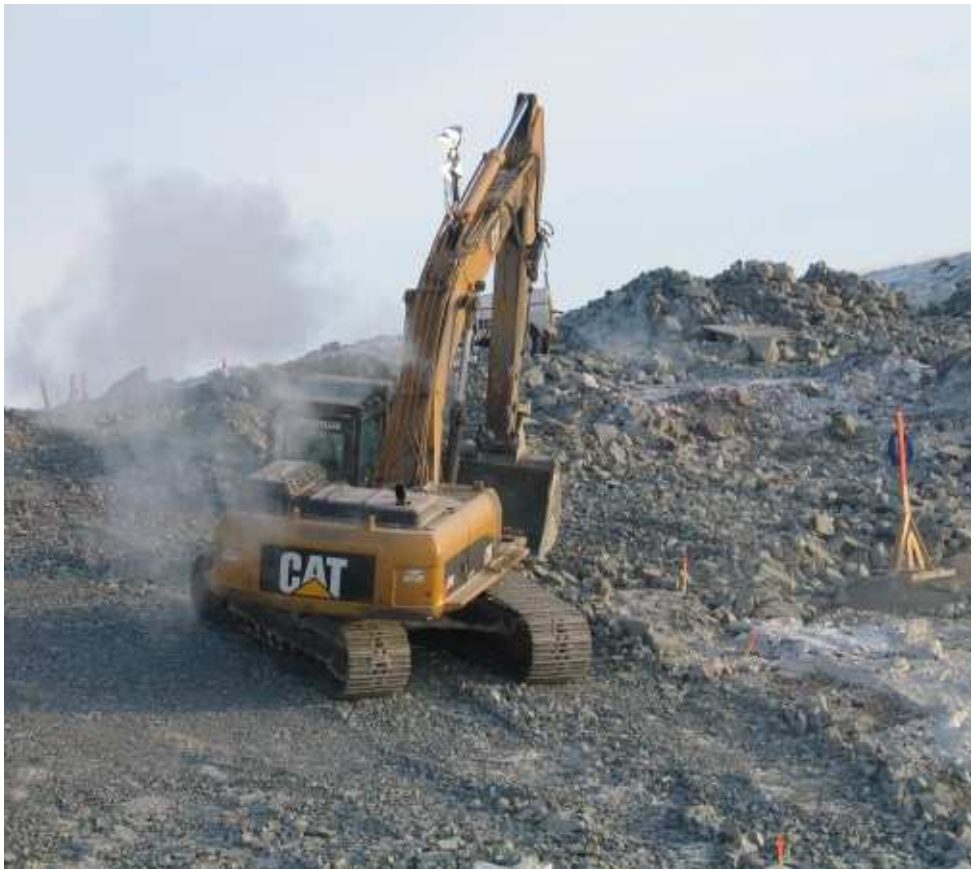
Photo 7: Excavator backsloping at Stn 0+40
