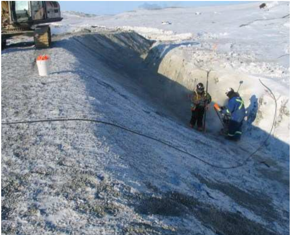
Photo 9: Surveying top of crush at Sta 3+30
